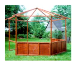
1. Start assembling the frame with the **corner posts** and **side panels**. First use two side panels to support the frame. Try not to twist the connector hinges, they might otherwise get blocked. Make sure the **side panels** are in the correct orientation, some might have hinges for the counter.
